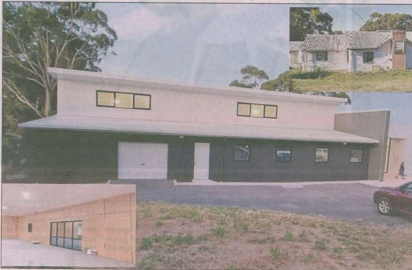
What a difference 15 months makes. The ribbon will be cut on the $1 million Ballan Scout hall with a community open day this Sunday. Pictures by Gabrielle Hodson.
